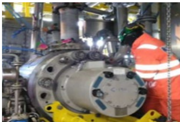
TEG export compressor bundle installation
