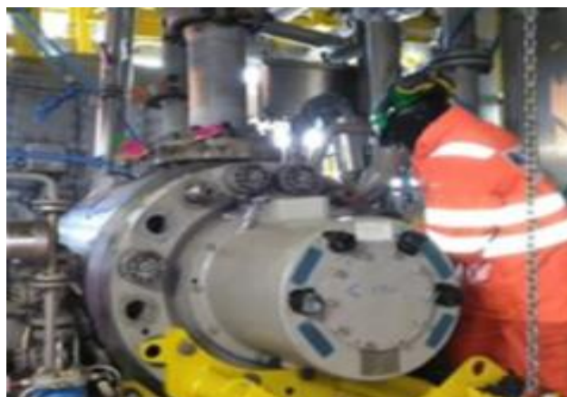
TEG export compressor bundle installation
