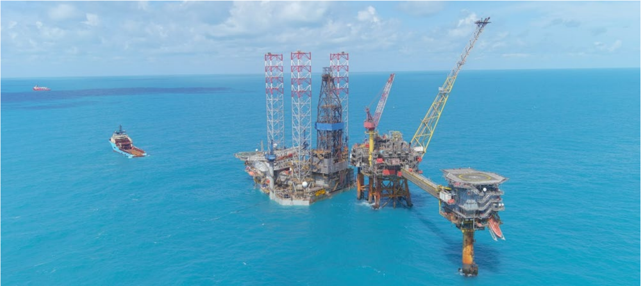
The rig Shelf Drilling Winner alongside the Harald platform to drill the Harald East Middle Jurassic Well
